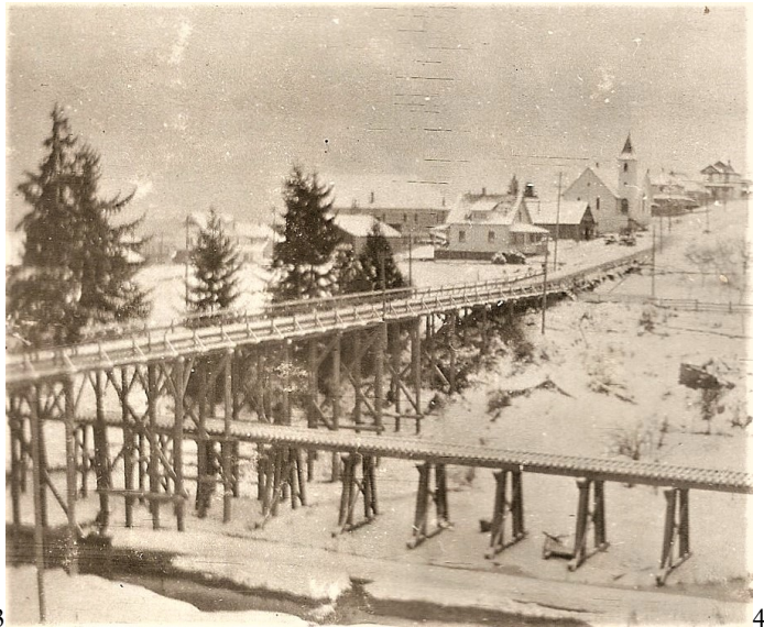
The photo at left, looking northwest, shows the Hammond elevated railroad track ending at the river where the logs were unloaded. The tank shown near the end of the track held fuel oil for the steam locomotives. Oil was used as the main source of fuel rather than wood or coal. The photo at right, looking eastward, shows the track going under the Fox Creek Bridge. The Methodist Church can be seen in the upper right. The school house sat west of the tracks (from where this photo may've been taken).
