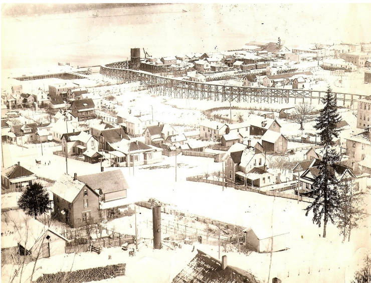
The photo at left, looking northwest, shows the Hammond elevated railroad track ending at the river where the logs were unloaded. The tank shown near the end of the track held fuel oil for the steam locomotives. Oil was used as the main source of fuel rather than wood or coal. The photo at right, looking eastward, shows the track going under the Fox Creek Bridge. The Methodist Church can be seen in the upper right. The school house sat west of the tracks (from where this photo may've been taken).
