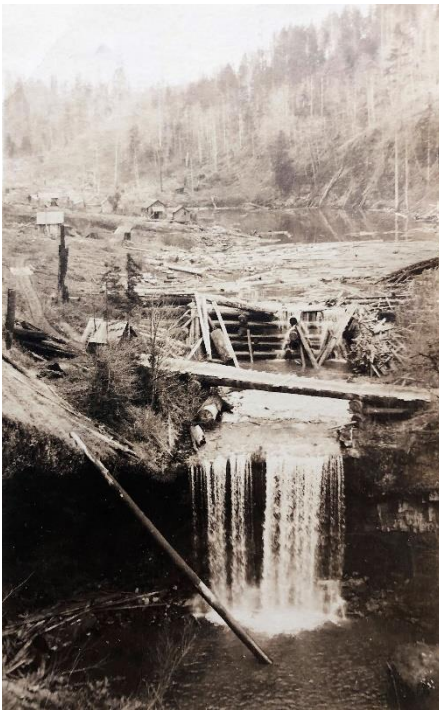
An example of a splash dam constructed at Beaver Falls.
